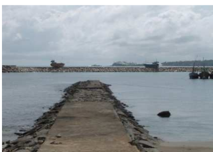
Hikkaduwa Fishery Harbour Reconstruction
