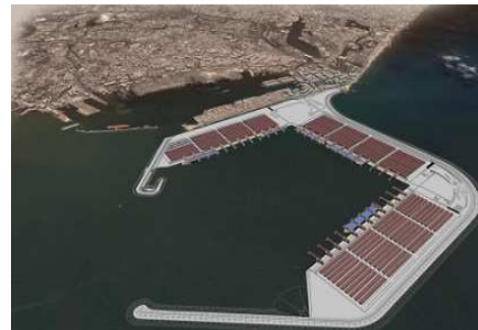
Colombo South Harbour Development
